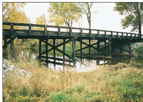
Pipe Creek Bridge
