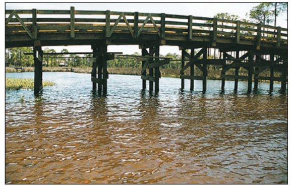
Horseshoe Bayou Bridge
