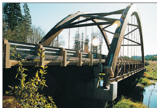
Dairy Creek Bridge
